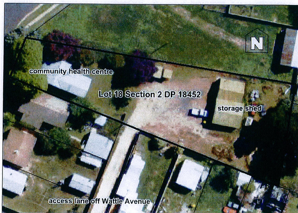
Photograph 1 Captains Flat Community Health Centre and works compound
